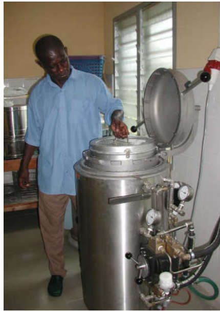
Fig. 2: Left: Second generation prototype of the autoclave as installed in a district hospital in Eikwe, Ghana.
